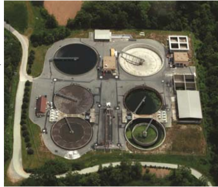
Little Falls Run WWTF - Stafford County, VA
