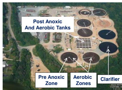
Aquia WWTF - Stafford County, VA
