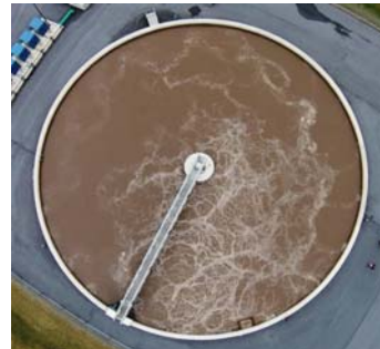
CSR Process with Rotating Bridge
